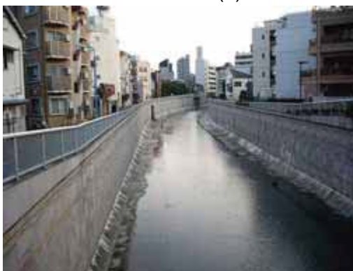
Restored with much concrete (1)
