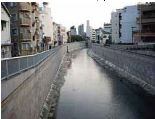
Restored with much concrete (1)
